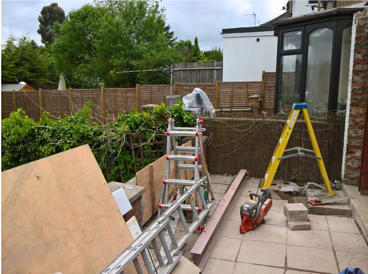
Rear conservatory and patio of No. 106 in background
